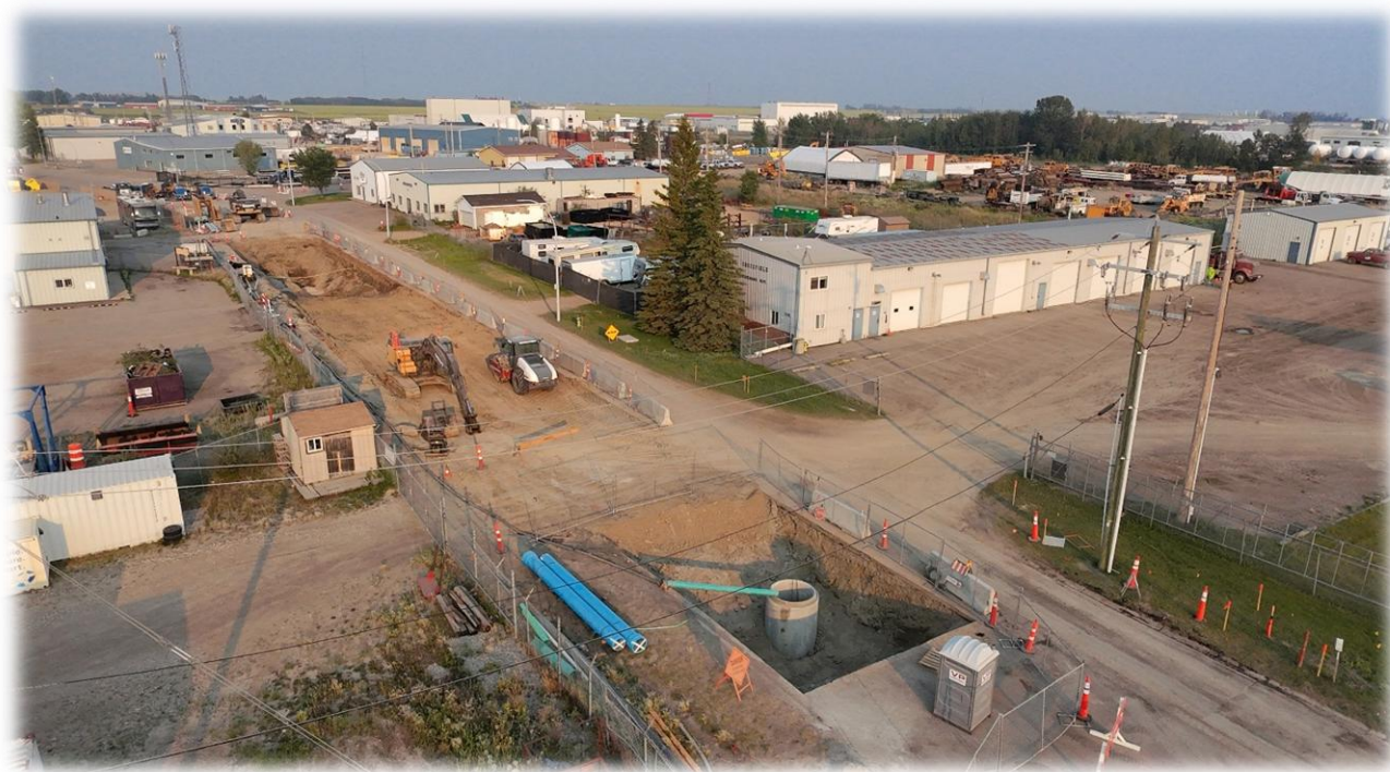
Construction progress along Laut Avenue - 2026
